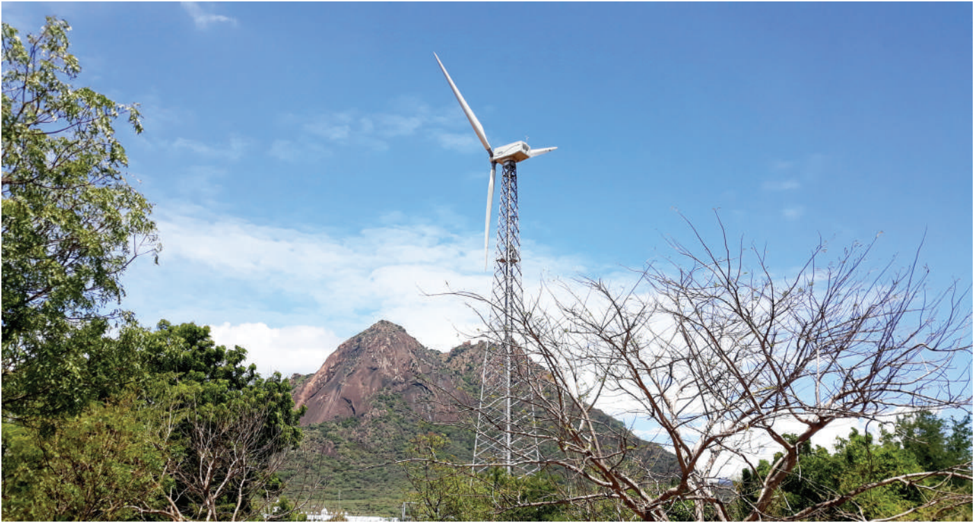
The five sites that CSE visited featured turbines that were more than 20 years old
