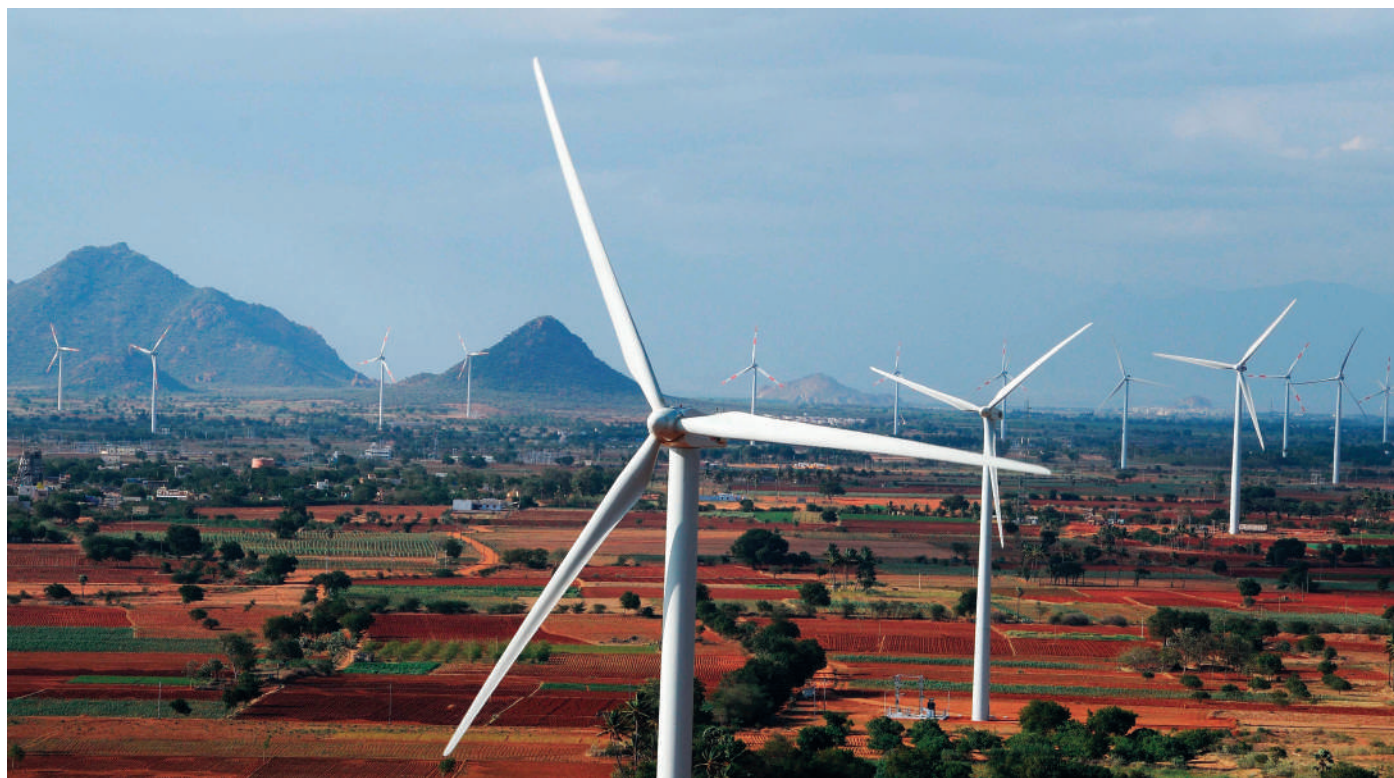
Dismantling and disposing of old turbine components, and other such activities, cost Rs 12 lakh for a 250-kW wind repowered project
