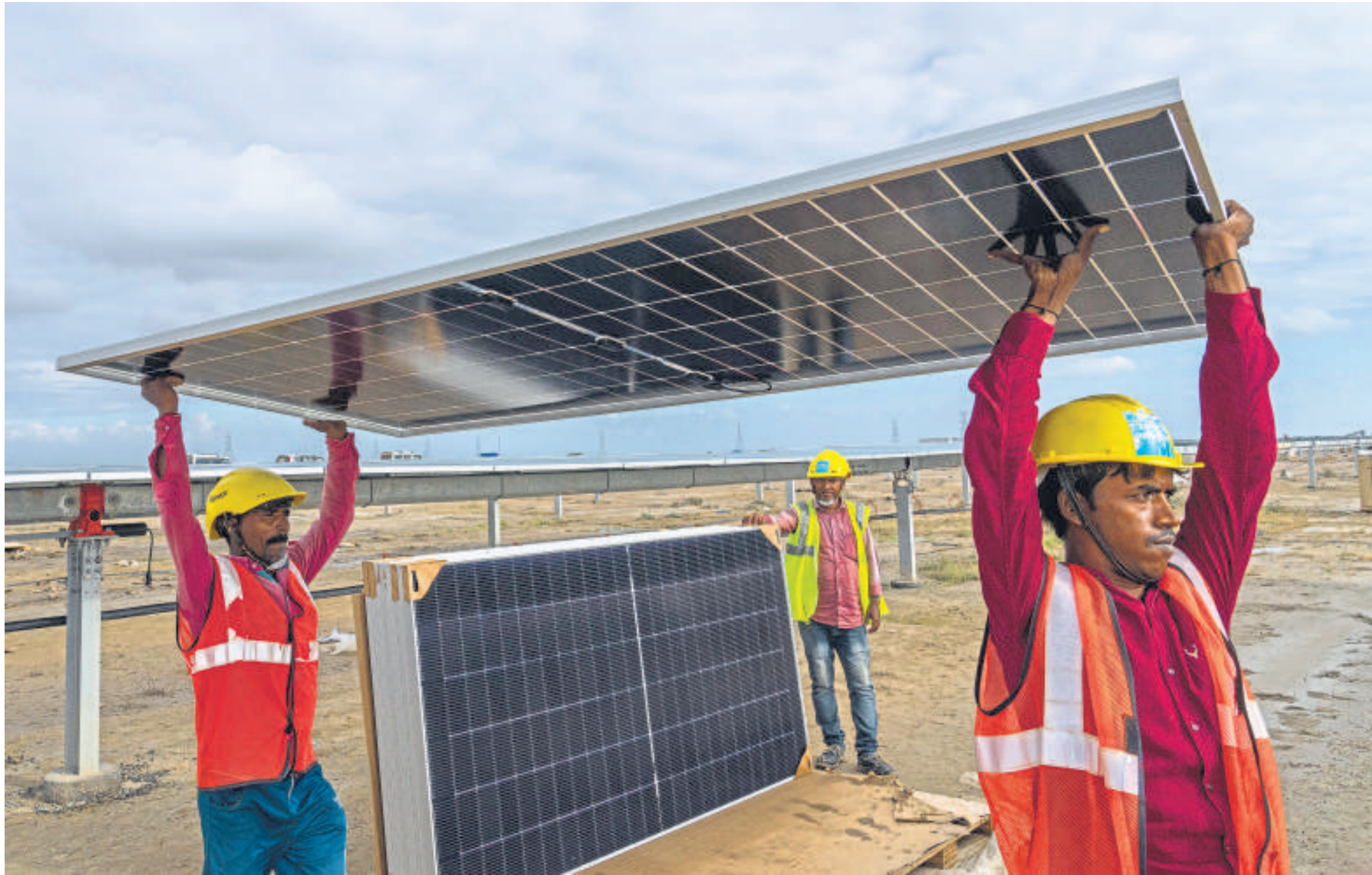
A file photo of workers carrying a solar panel for installation at an under-construction renewable energy project in Gujarat's Kutch district.
